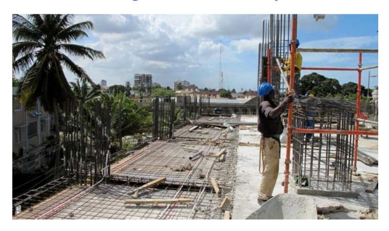
Edge protection will be required at the edge of floor openings and stairs, and wherever there is a drop of 2m or more
