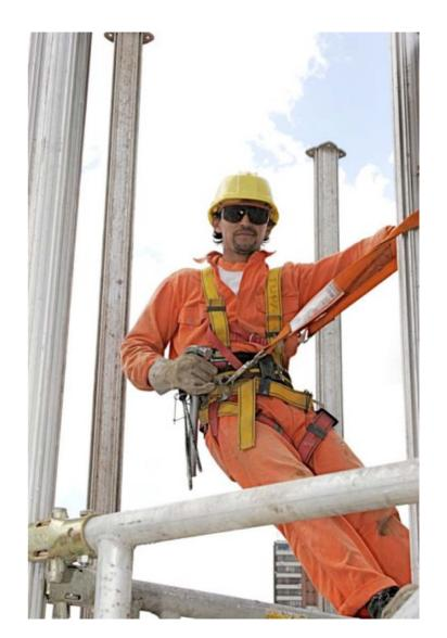
The photo shows an alternative form of harness, attached at the back.
