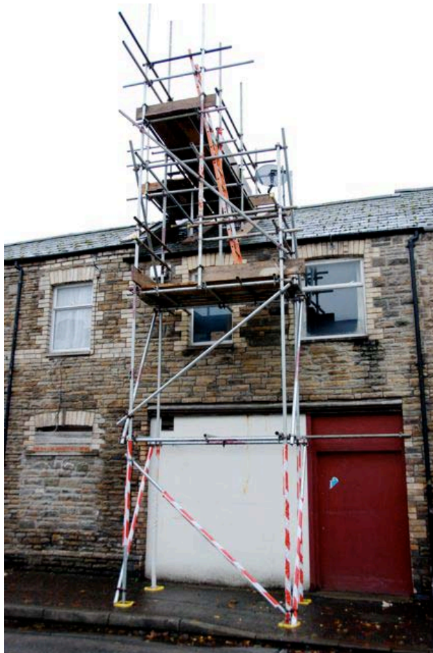
(Photo: Richard Neale, permission granted by the scaffolders)
