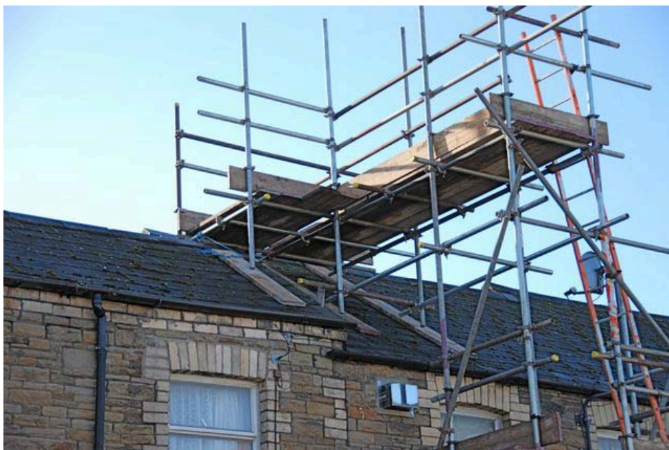
(Photo: Richard Neale, permission granted by the scaffolders)
