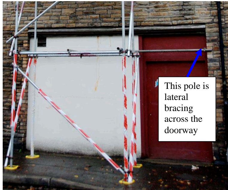
(Photo: Richard Neale, permission granted by the scaffolders)
