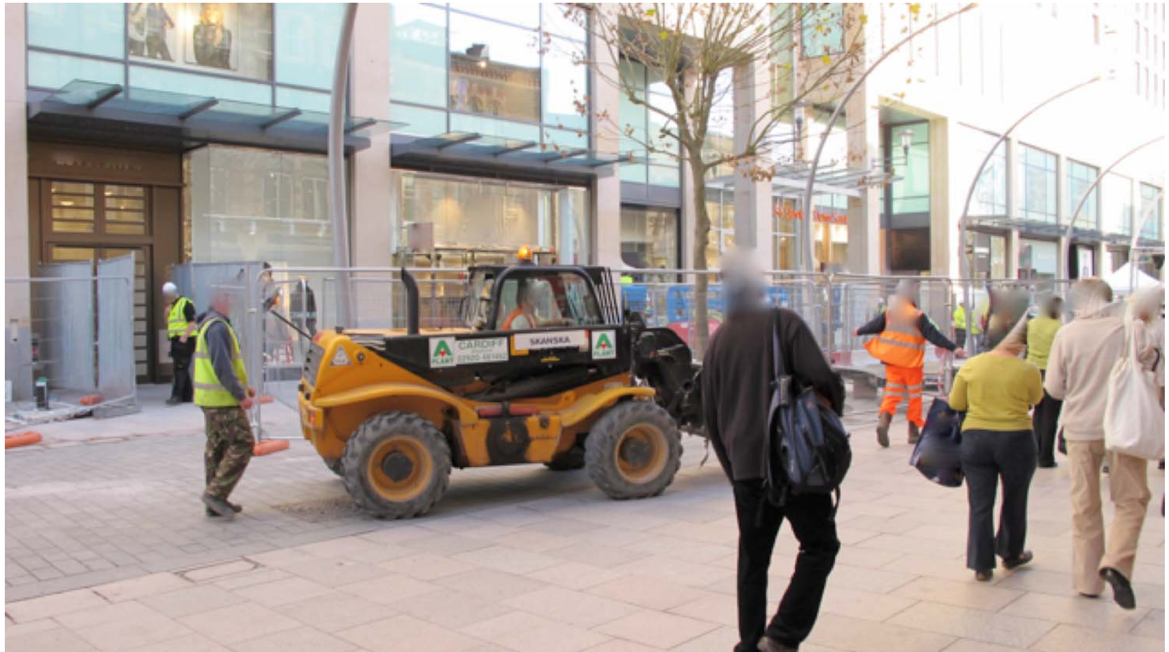
The photo shows two banksmen escorting a vehicle in a busy street.
