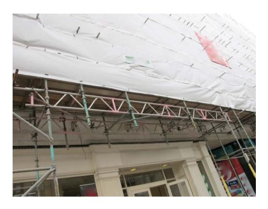
A beam is necessary over shop doorways and this is attached by conventional tube and fittings.
