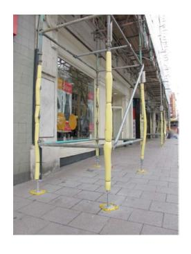
The uprights are encased in highly visible plastic foam to prevent damage to passing pedestrians.
