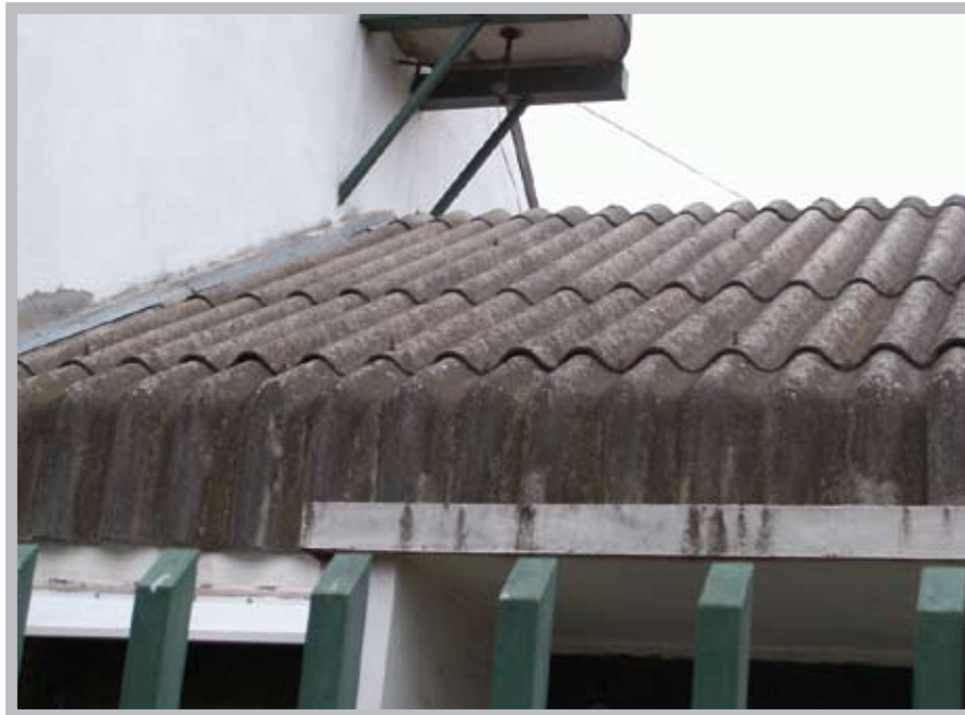
Single-family house with fibrous cement plates
