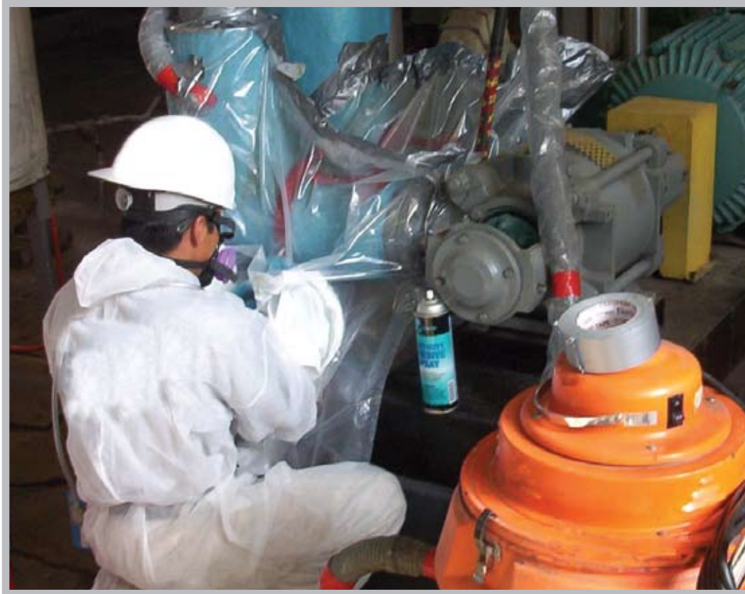
Removal with GLOVEBAG system
