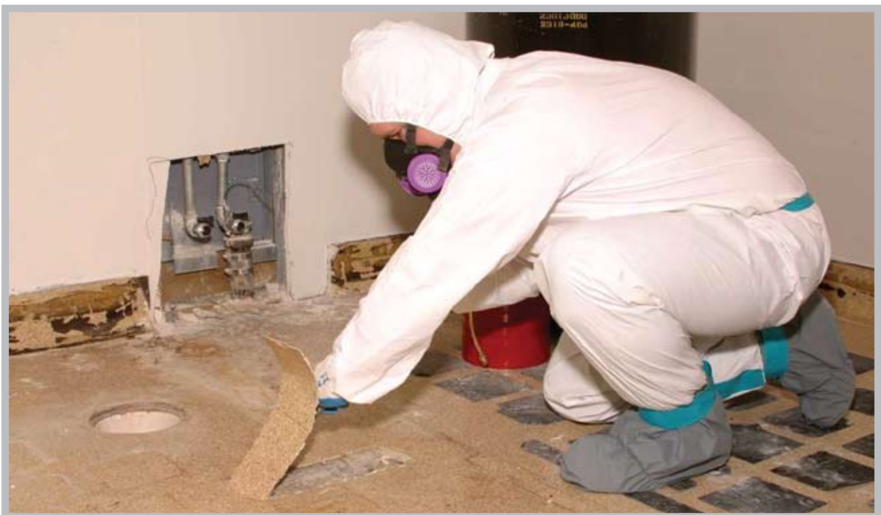
Asbestos Removal
