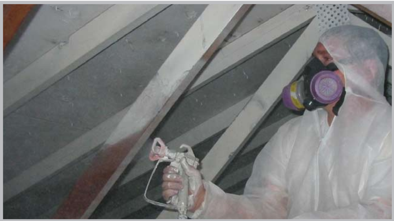
Asbestos Encapsulation
