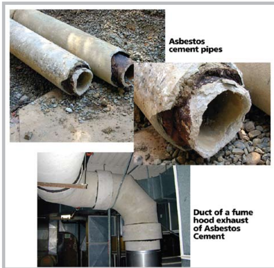
Asbestos cement pipes
