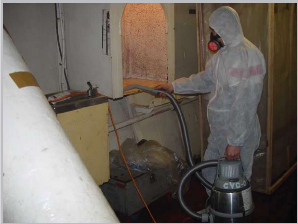
Removal of asbestos dusts
